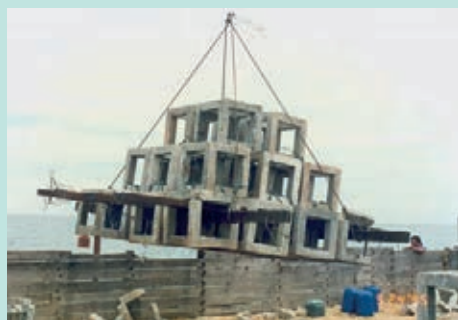
Twenty nine unit recreational concrete ARs deployed in Pulau Rhu, Terengganu
