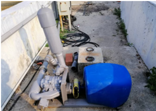
Gambar 16 : “ Blower super charger ” (2hp)
