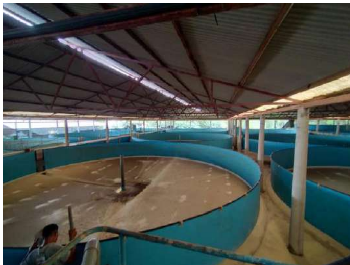
Figure 2: Indoor RAS system will ensure the sustainable operation regardless the effect of monsoon season in tropical country, including Malaysia.
